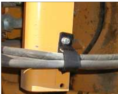
Hanging strap is used to bundle and support the hoses
