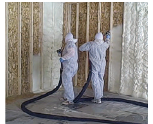
Radiant-lined 5601 helps maintain chemical viscosity in the spray foam industry.
