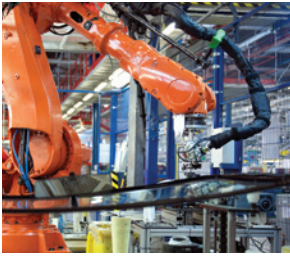
Bundle and protect critical cables and wires near engine turbo compartments.
